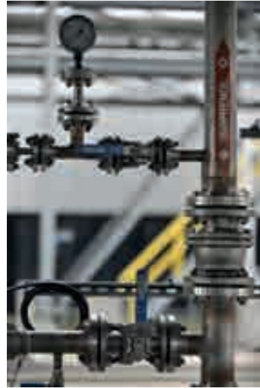
© Gilles Dacquin – Transfer pipe for chemical products
