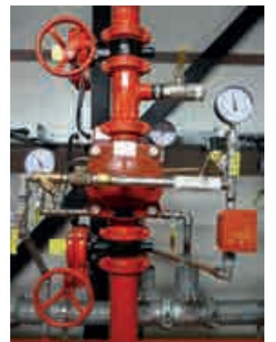
Fire system valves.
